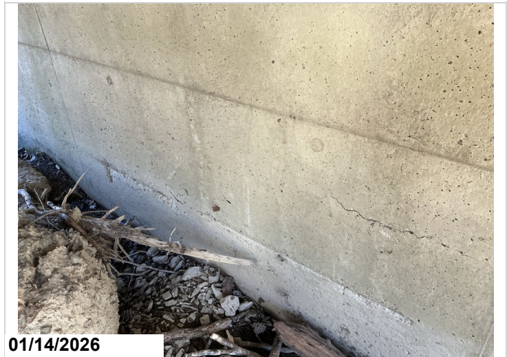
Bent 2: the entire length of the abutment has exposed rebar and honey combing.
