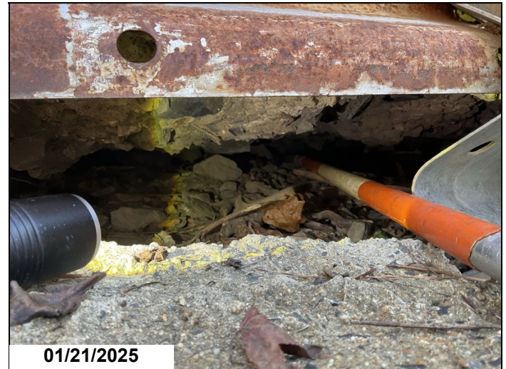
Northwest corner of bridge, approach slab is undermined 8' under roadway. Void is approximately 8" deep
