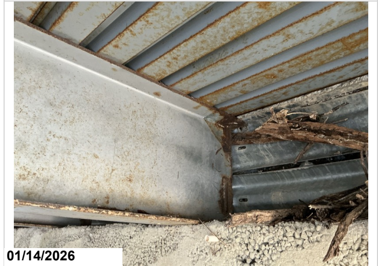
Bent 2, girder 4: girder ends with small amount of active rust. This is common to all girders ends at both bents.
