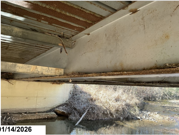
All girders have areas of freckling rust.
