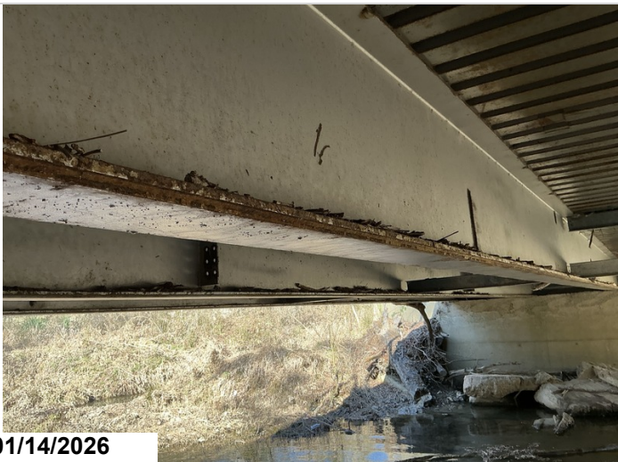
All girders have scattered areas of corrosion.
