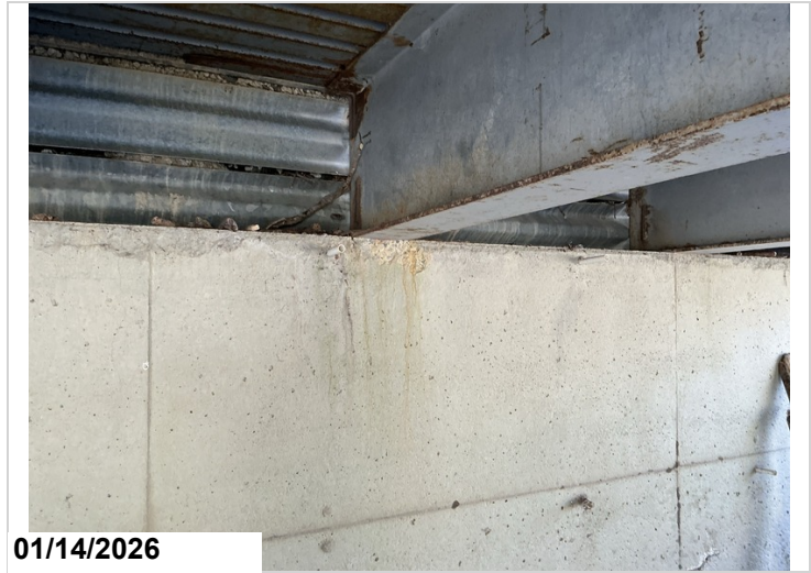
Bent 1 spall under girder 3.
