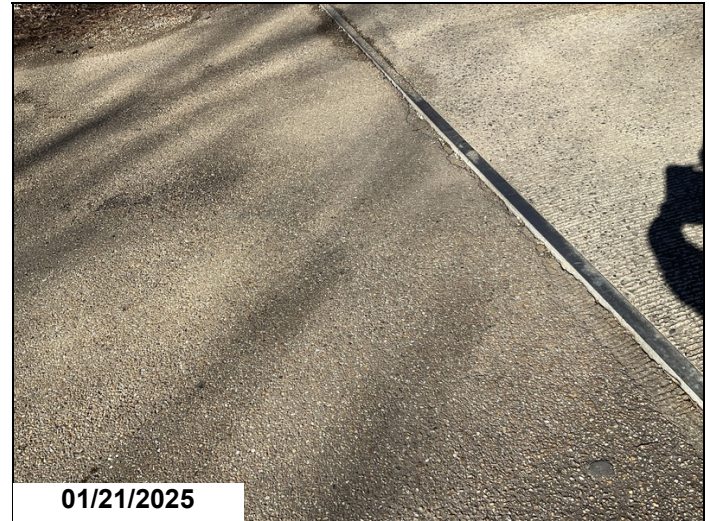
Bent 1 approach slab has settled 1". Approach slabs is undermined up to 3' by 8" deep.
